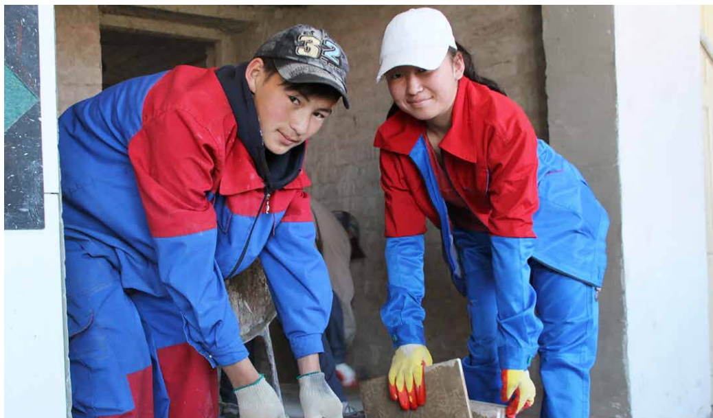
Mason apprentices at work in Mongolia
