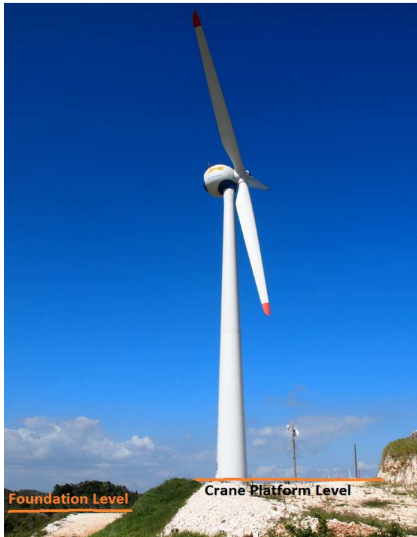
Figure 2-19: Crane Platform and Foundation Level showing approx 2 m Difference in Elevation
