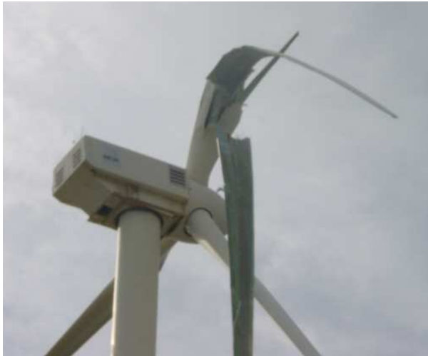
Figure 2-139: Rotor Blade Damage due to Lightning Strike
