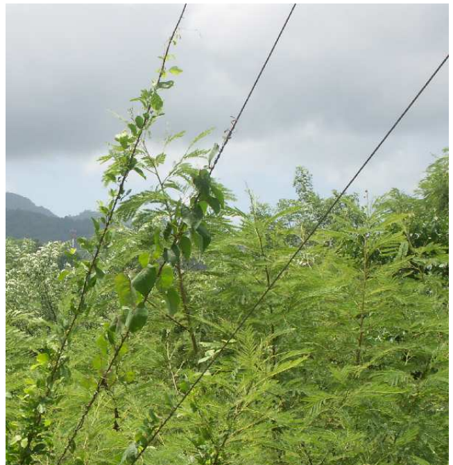
Figure 2-59: Lake Antoine, Guy Wires Measuring Tower
