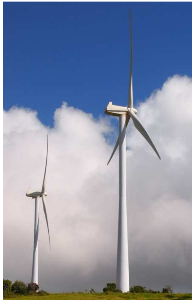
Figure 2- 1: NEG Micon NM52 - 900 kW Wind Turbine at Wigton, Jamaica
