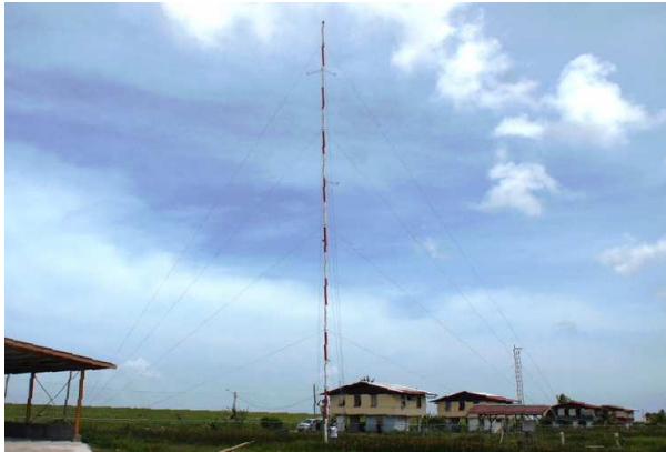
Figure 2-30: Micro-Location of the 30 m Wind Measuring Tower – Nieuw Nickerie
