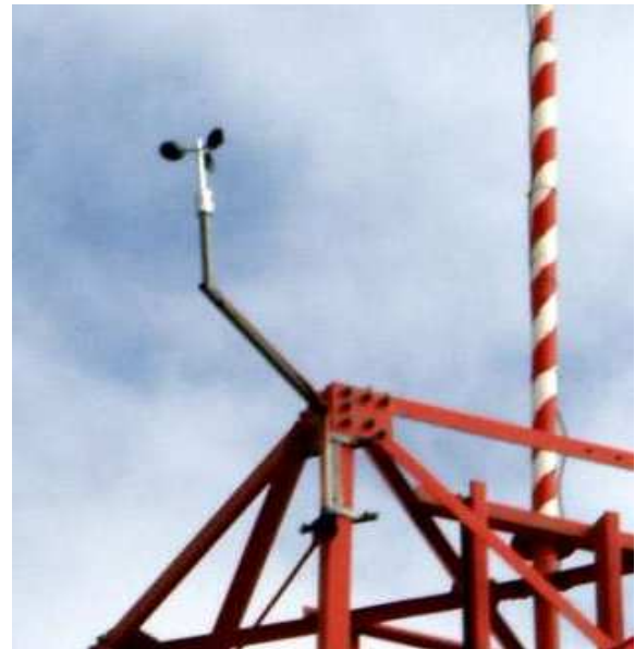
Figure 2-23: Example of Anemometer being Mounted to an existing Telecommunication Tower
