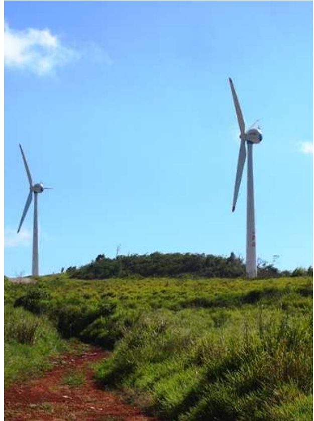
Figure 2-18: Munro Wind Park – Western Group
