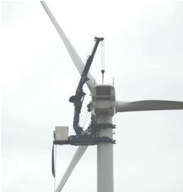
Figure 2-154: “Climber” Crane for Exchange of Gearbox
