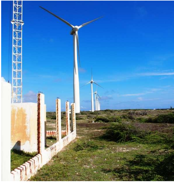
Figure 2-142: Fence around the Substation - Stolen
