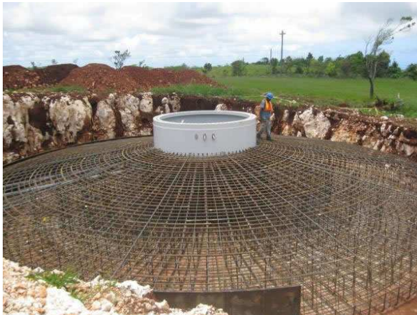
Figure 2-7: Wigton II - Construction of Foundation for Vestas V80 – 2 MW
