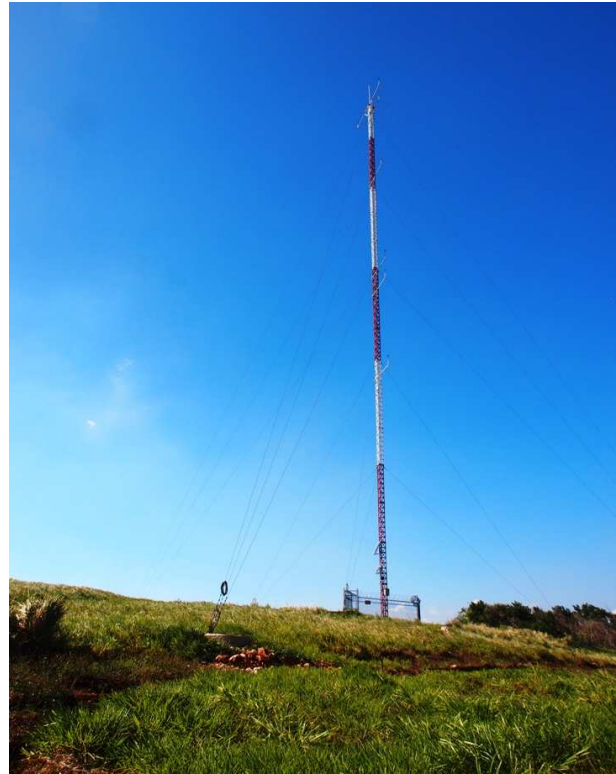
Figure 2-20: Munro Wind Park 50 m Measuring Tower for Expansion
