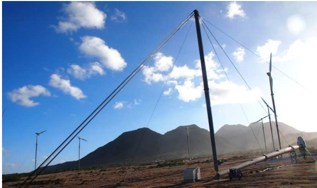
Figure 2-106: Maddens Wind Park with One Turbine Down for Maintenance
