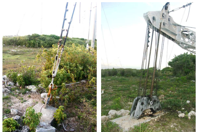
Figure 2-83: Guy-Wires and Tilting Mechanism/Gin Pole
