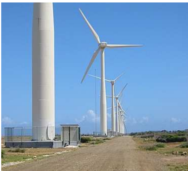
Figure 2-143: Original Fencing around the Foundation (2002)
