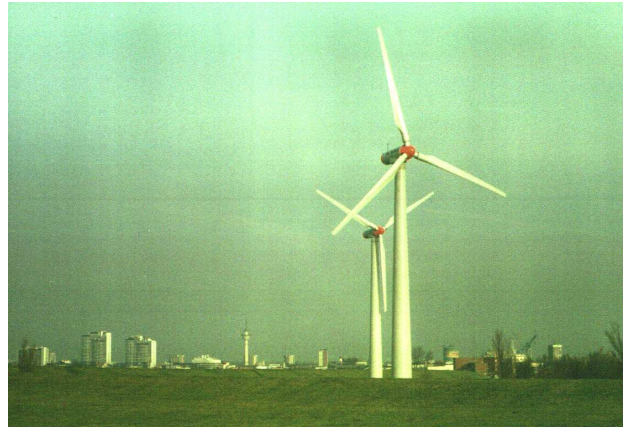
Figure 2-32: Wind Turbines behind Dyke (Bremerhaven)
