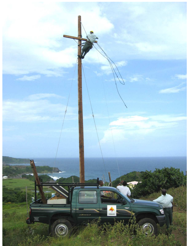
Figure 2-88: Installation of Anemometer Station at Brighton
