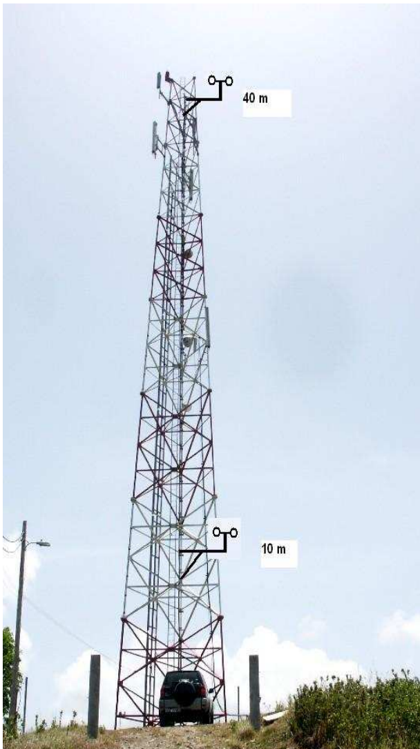
Figure 2-99: Antennae Tower at Maddens Estate with two proposed Anemometers
