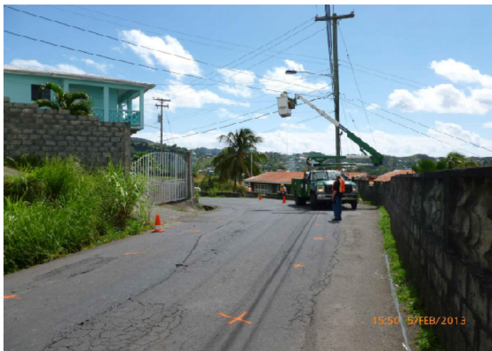
Figure 5: Test road at Questelles
