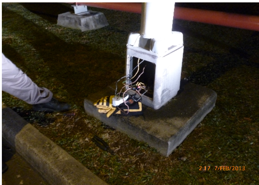
Figure 6: Arrangement to measure the electrical parameters
