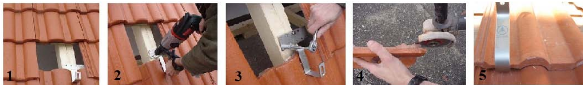
Figure 5.10: Tile hooks mounting, source: Schletter GmbH
