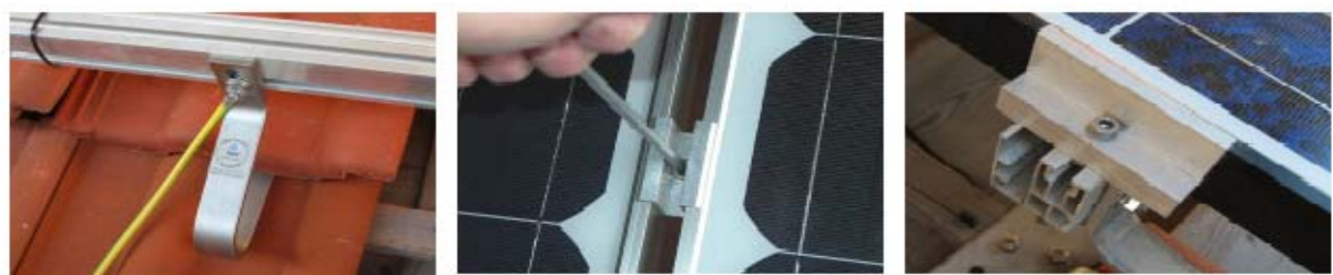
Figure 5.11: Beam-tile hooks attachment, module mounting, Source: www.solarzentrum-allgaeu.de
