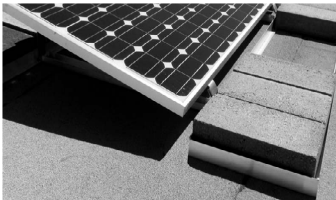
Figure 5.7: Flat roof mounting, source: www.unirac.com
