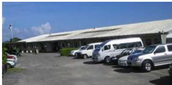
Ministry of Agriculture Building, Graeme Hall, Barbados where the first Solar AC installation in the Region was located
