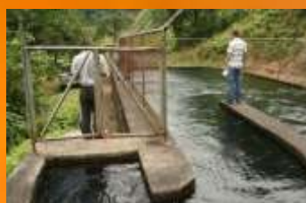
South River Hydro Project, St. Vincent & the Grenadines
