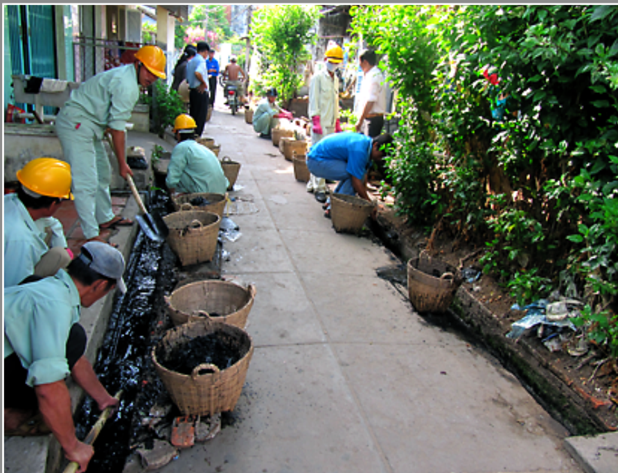
Cleaning tertiary sewer system (cleaning campaign), Tra Vinh, 02.06.2010
