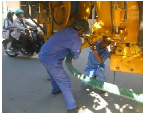
Practicing sewer cleaning by suction vehicle in Can Tho.
