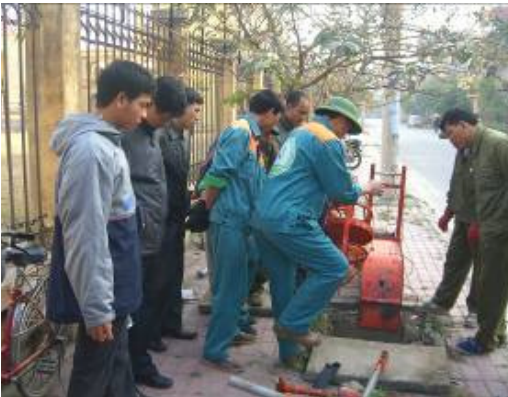
Practicing sewer cleaning by winch system in Hai Duong
