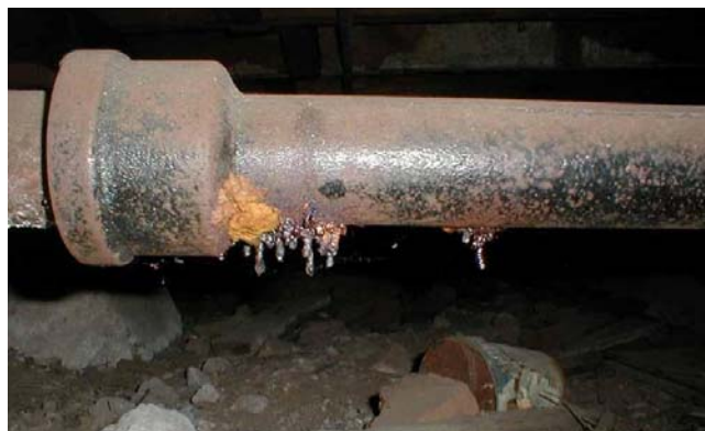
Figure 3: Photo of pipe inspection activity
