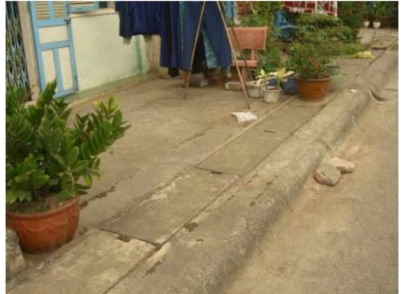
Photo 10: Public drain – Ward 9
