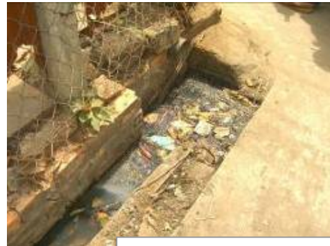
Tertiary sewer at Ward 7
