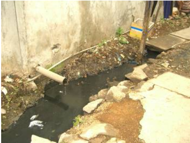
Photo 3: Natural ditch to which household wastewater is discharged – Ward 2
