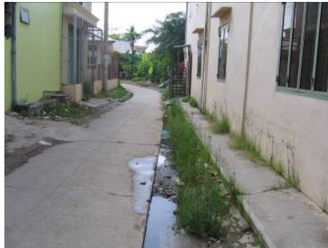
Photo 5: Natural ditch to which household wastewater is discharged – An Nghiep Ward
