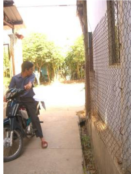
Photo 2: Public drain – Ward 1
