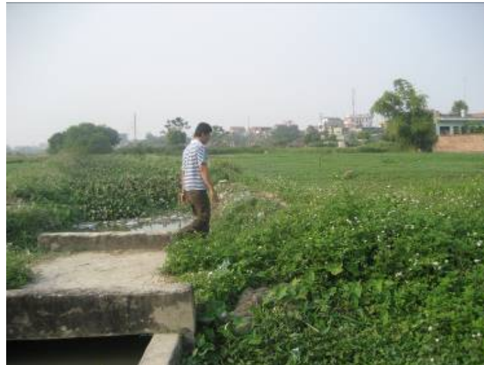
Photo 3: Channel discharge wastewater to land field – Ve An Ward
