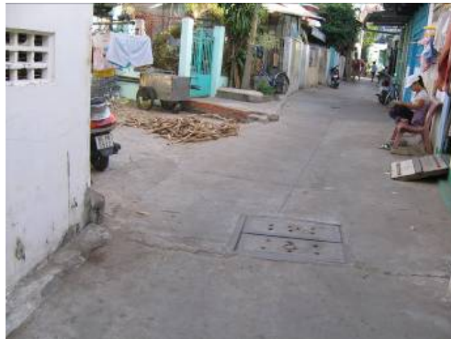
Photo 3: New public drain installed by World Bank Bank Project – An Cu Ward
