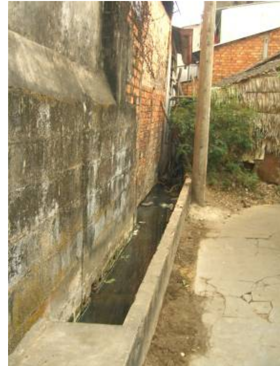
Photo 4: Public drain – Ward 2
