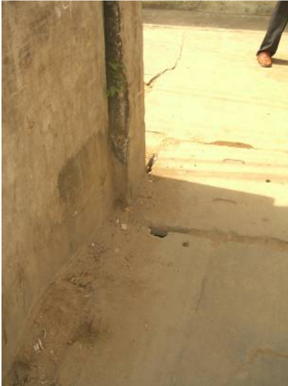
Photo 3: Public drain – Ward 2
