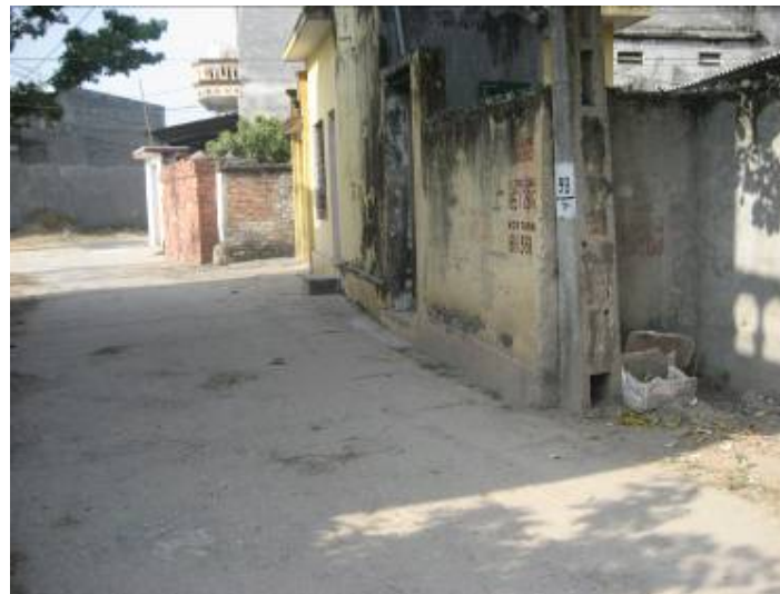
Photo 9: Part of tertiary drain - Vu Ninh Ward
