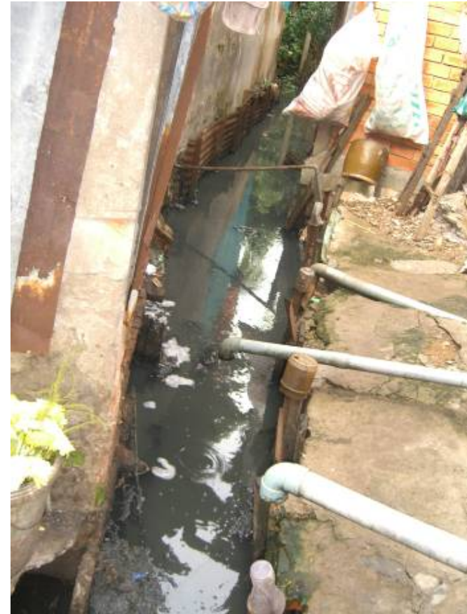
Photo 9: Natural ditch to which household wastewater is discharged – An Lac Ward
