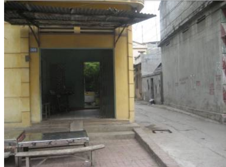
Photo 2: Part of tertiary drain - Ve An Ward
