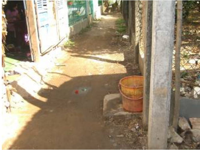
Photo 1: Lane where PVC pipe is laid for discharging household wastewater – Ward 1
