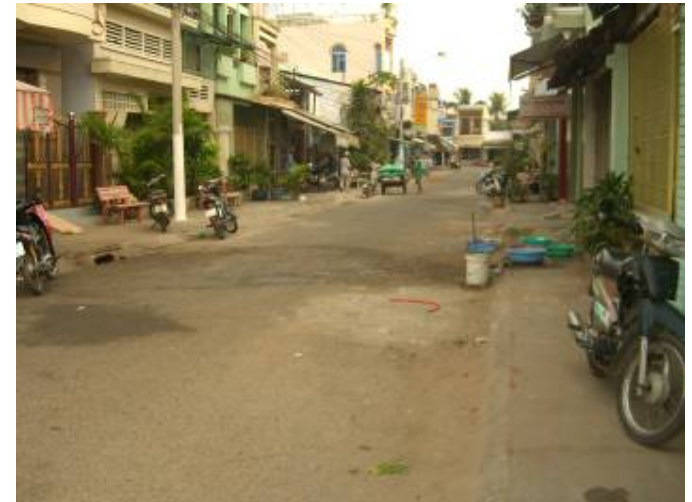
Photo 8: Public drain – Ward 6
