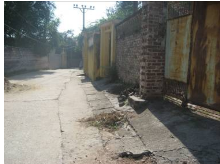
Photo 11: Public drain – Dap Cau Ward
