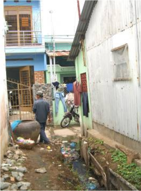
Photo 1: Natural ditch – Ward 1
