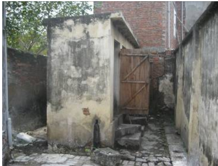
Photo 6: Public toilet – Tien An Ward
