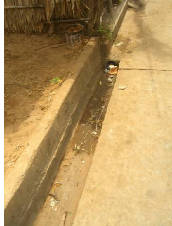
Photo 4: Public drain – Ward 2
