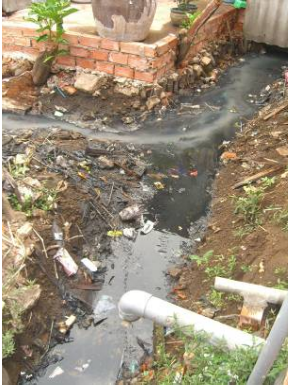
Photo 5: Natural ditch to which household wastewater is discharged – Ward 3
