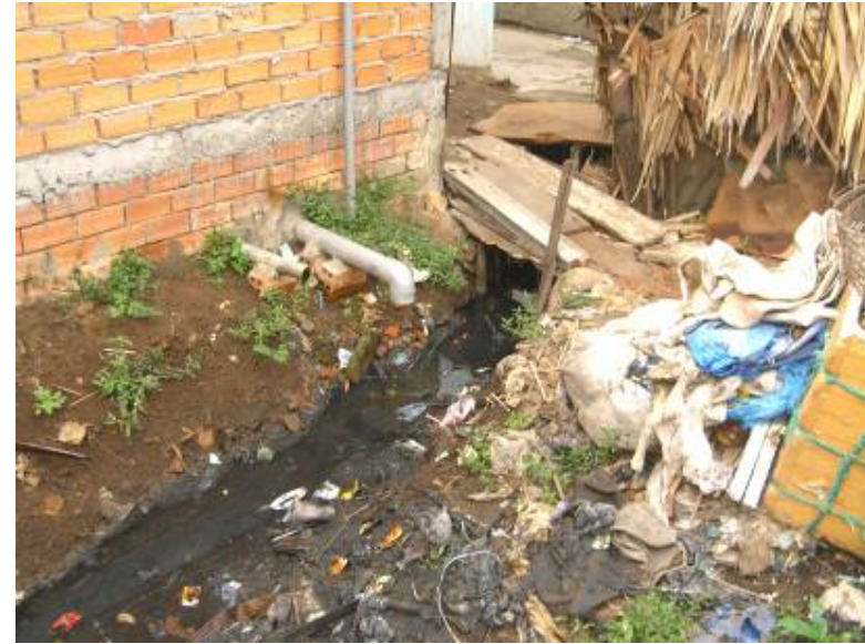
Photo 6: Natural ditch to which household wastewater is discharged – Ward 3
