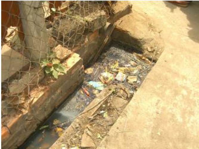
Photo 5: Public drain – Ward 7
