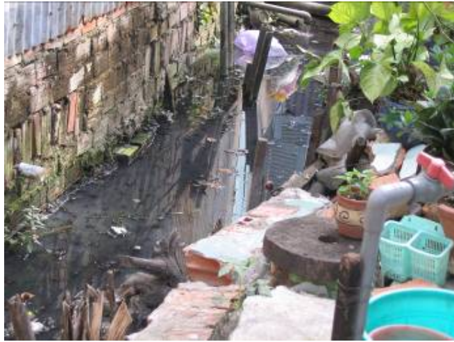
Photo 1: Natural ditch – An Cu Ward
