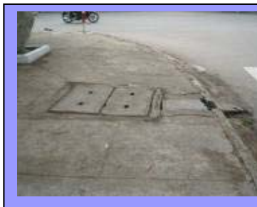
The covered drain in the main street
