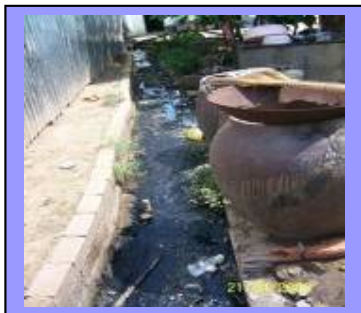
The open drain in an alley
