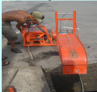
Positioning winch next to the manhole
