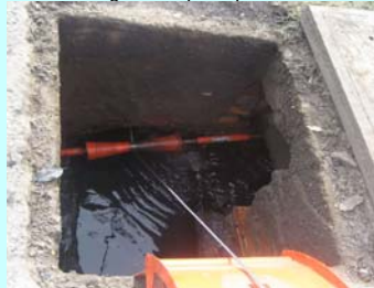
Positioning of direction-changing devices
