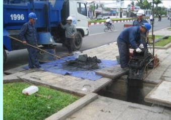
Remove sludge from sewer
