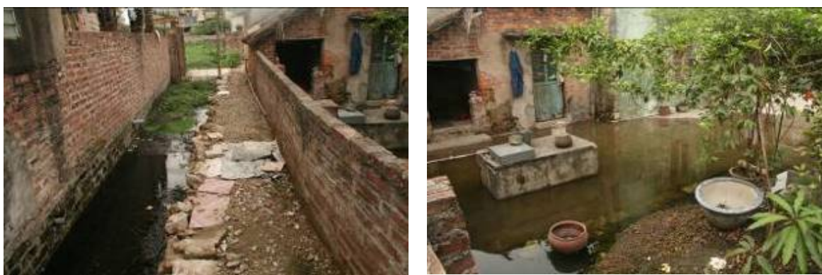
Figure 5-6 Public drainage system blockage in Binh Han Ward
