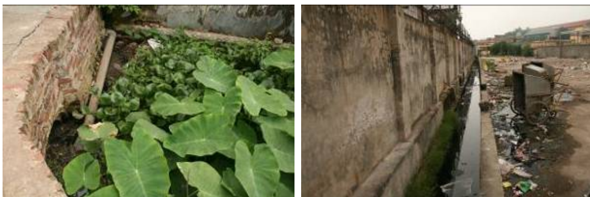
Figure 5-6 Public drainage system blockage in Binh Han Ward
