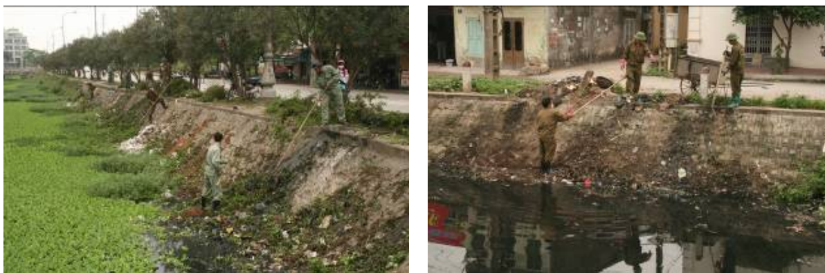
Figure 5-9 Company staff try hard to remove all waste and duckweed from canal T2 to the bank and then transport it to a landfill
